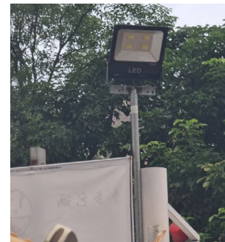
“Jiaxue.” Project Construction Site Fully Equipped with LED Lighting
